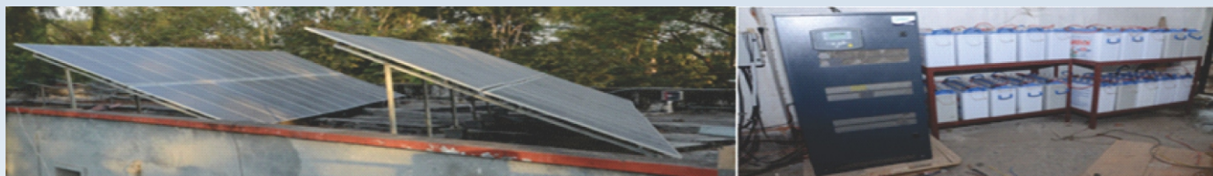
16 kW solar PV power-grid interactive system
